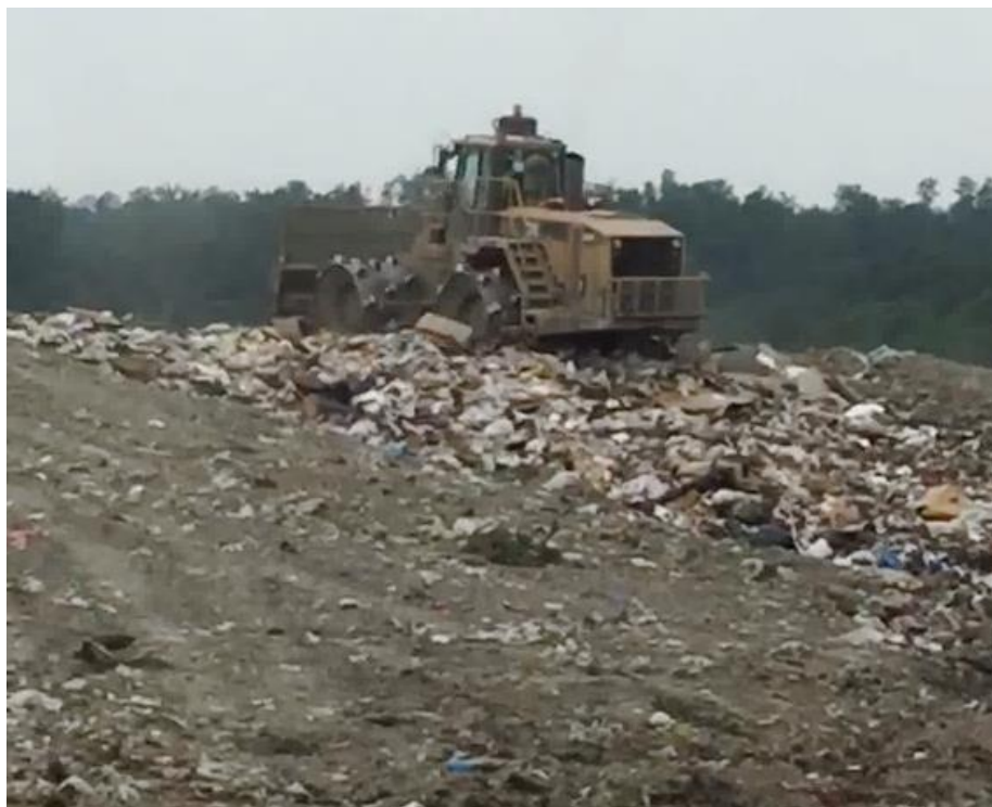
Figure 3. Compactor unit in the process of compacting disposed waste.
