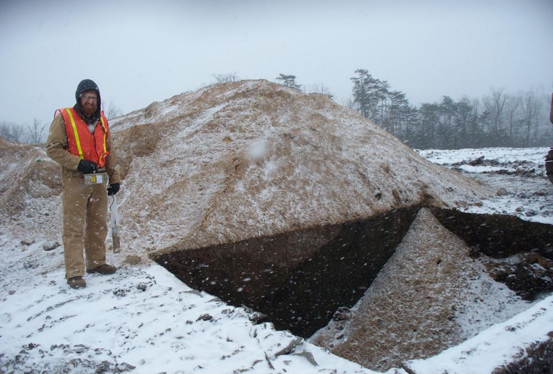
Advanced Disposal Blue Ridge Landfill AI 998 2/10/16 g. weems solidification pit. Testing for TENORM here since the TENORM was in sludge that had to be solidified prior to disposal.
