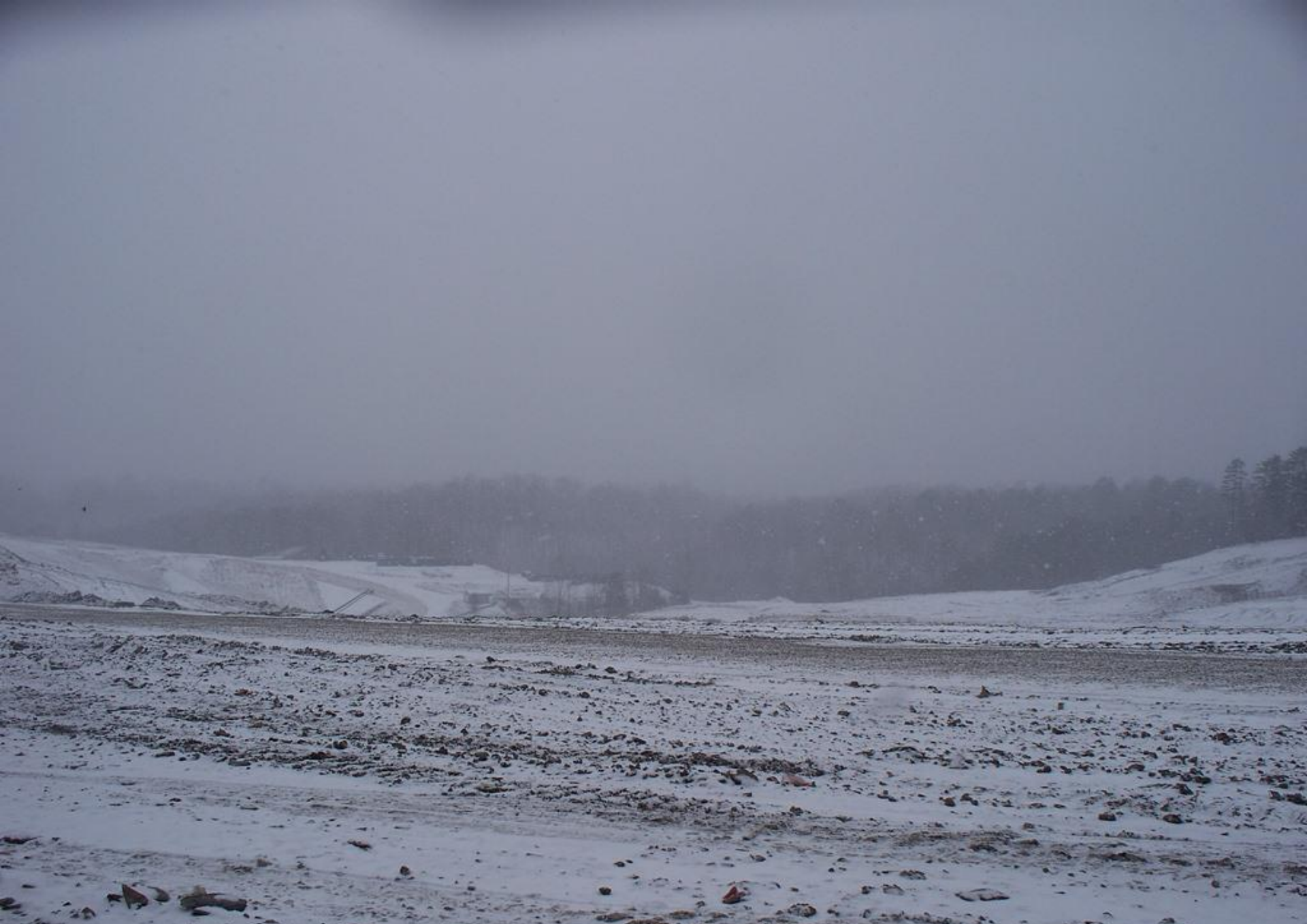
Advanced Disposal Blue Ridge Landfill AI 998 2/10/16 g. weems access road to working face
