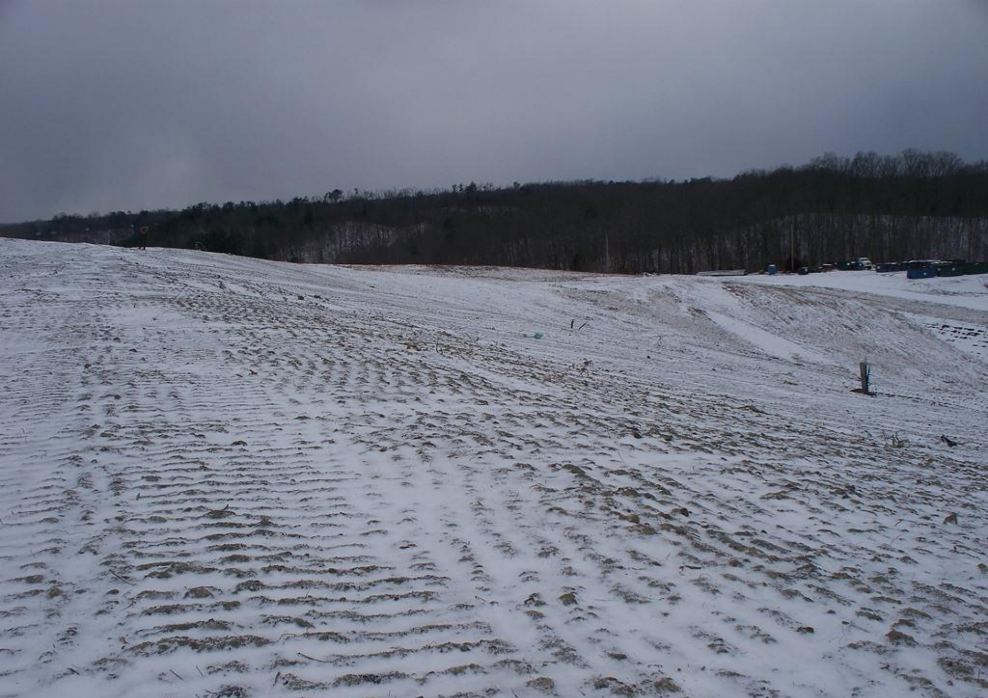
Advanced Disposal Blue Ridge Landfill AI 998 2/10/16 g. weems North side of working face.
