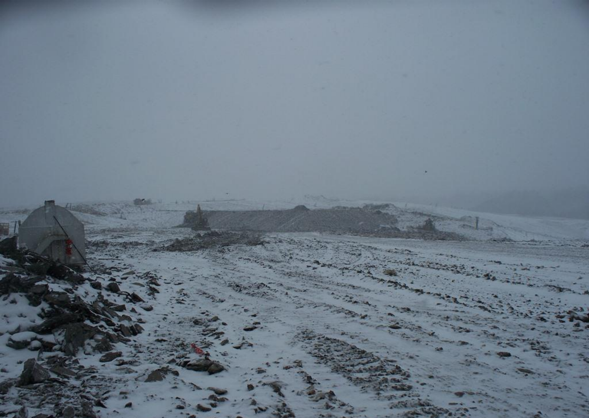
Advanced Disposal Blue Ridge Landfill AI 998 2/10/16 g. weems Looking toward working face
