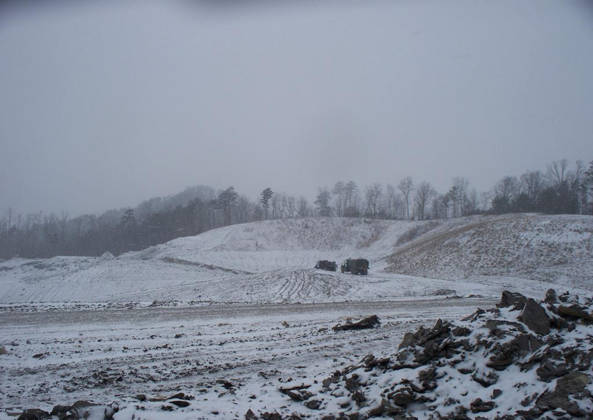
Advanced Disposal Blue Ridge Landfill AI 998 2/10/16 g. weems Borrow area
