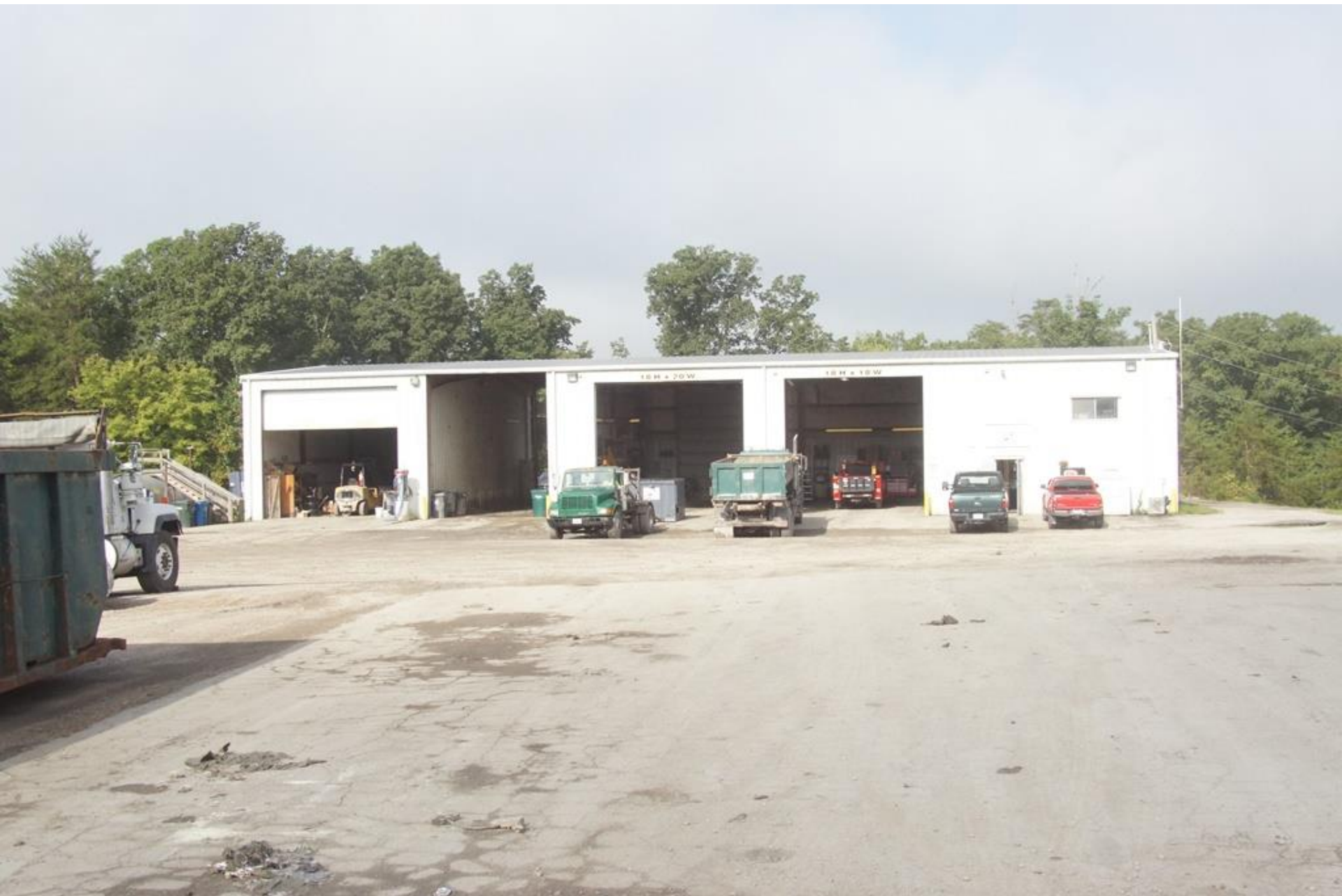
Advanced Disposal Blue Ridge Landfill AI 998 9/11/15 g. weems Maintenance building.
