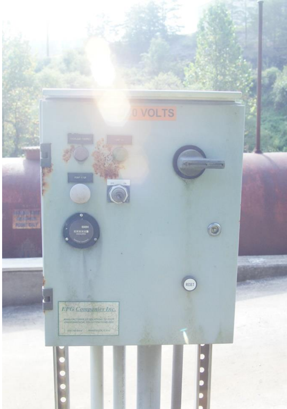
Advanced Disposal Blue Ridge Landfill AI 998 9/11/15 g. weems
