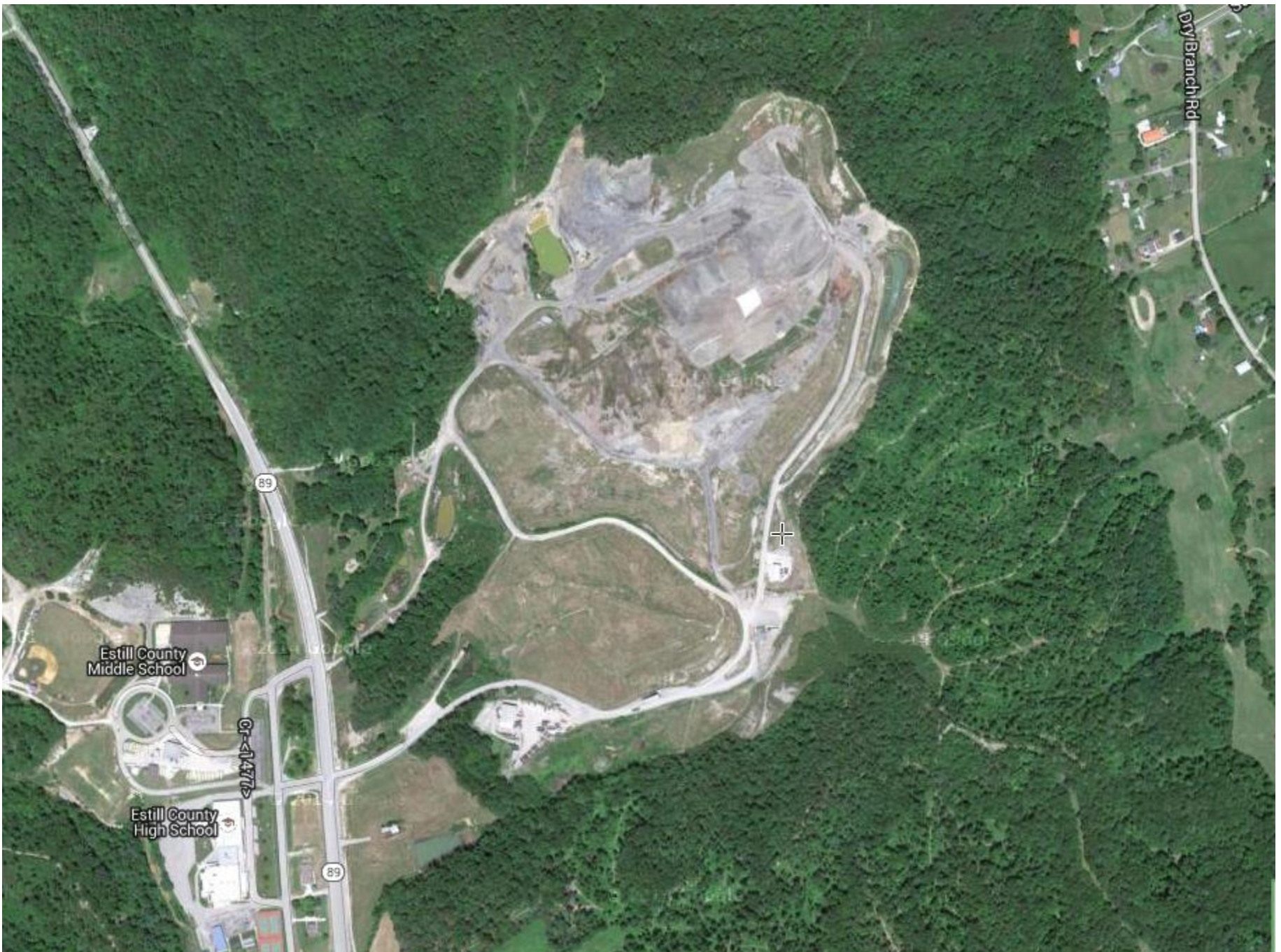
Advanced Disposal Blue Ridge Landfill AI 998 9/11/15 g. weems
