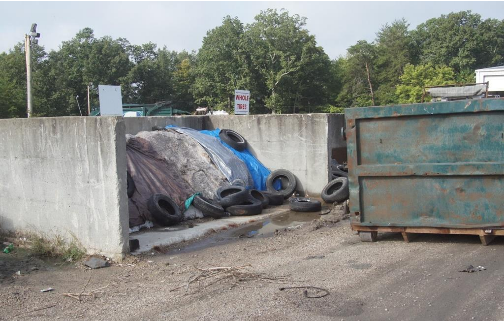
Advanced Disposal Blue Ridge Landfill AI 998 9/11/15 g. weems Tire pit in back. Front tires holding down cover.
