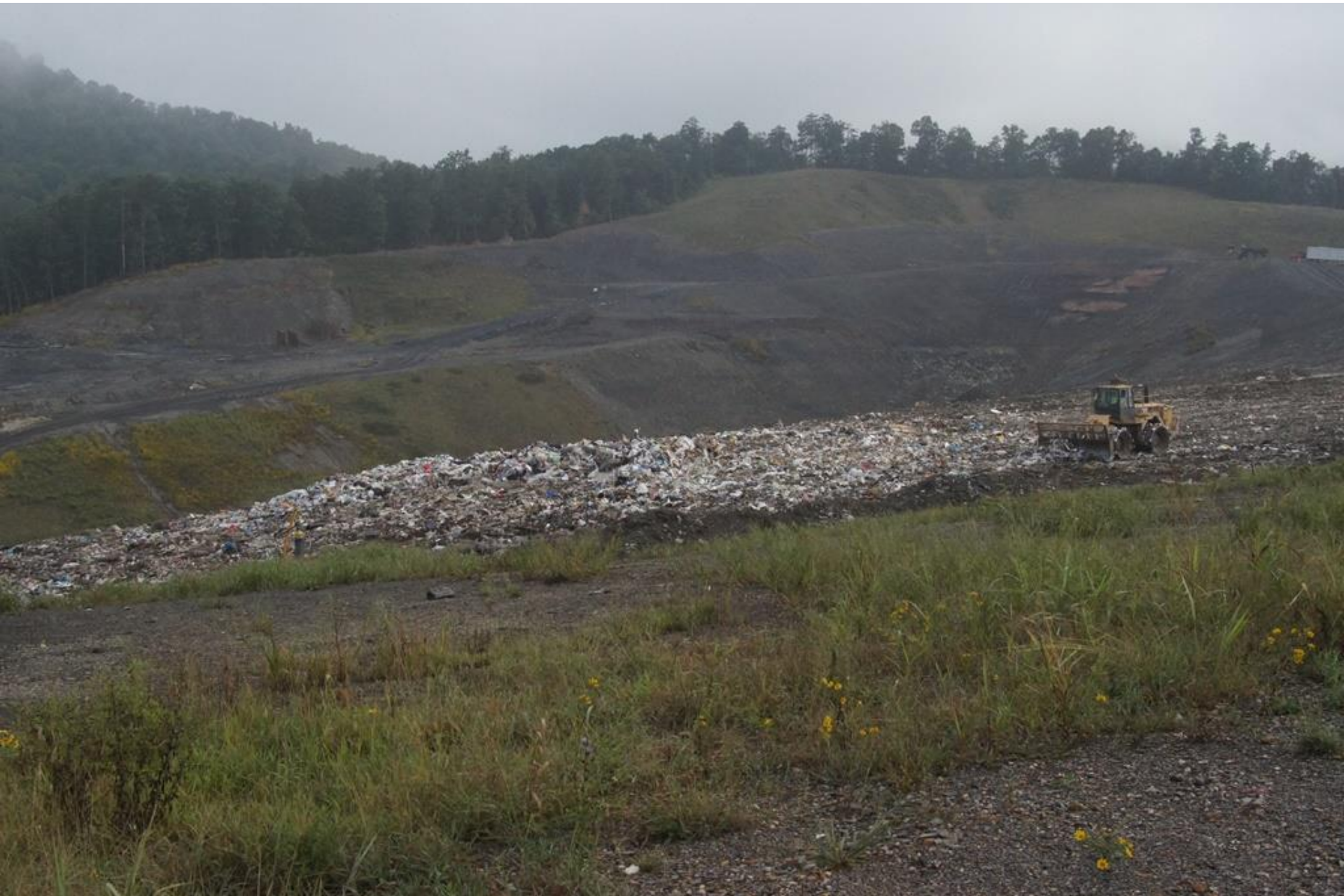
Advanced Disposal Blue Ridge Landfill AI 998 9/11/15 g. weems Working face
