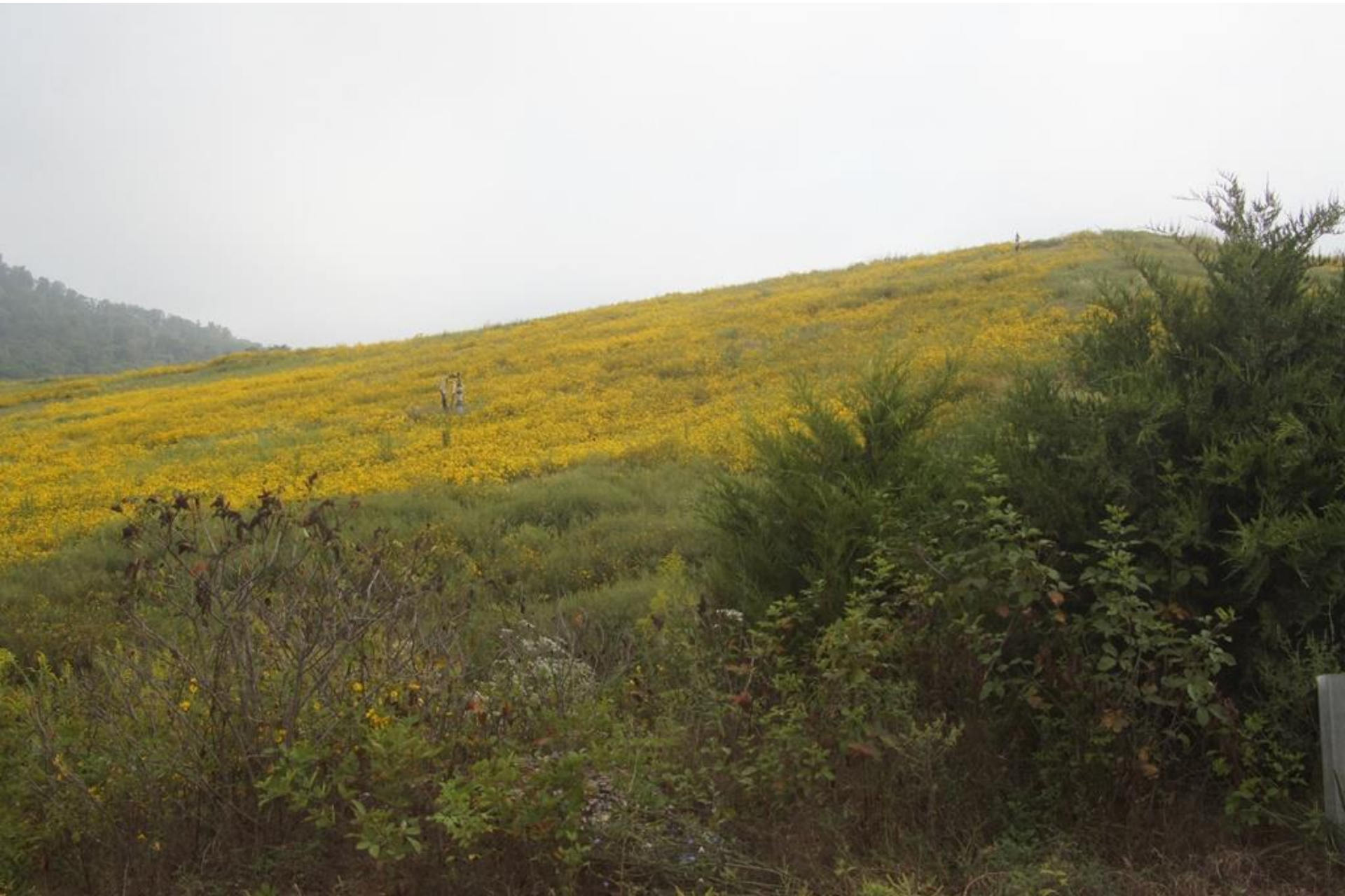
Advanced Disposal Blue Ridge Landfill AI 998 9/11/15 g. weems Cover is well established
