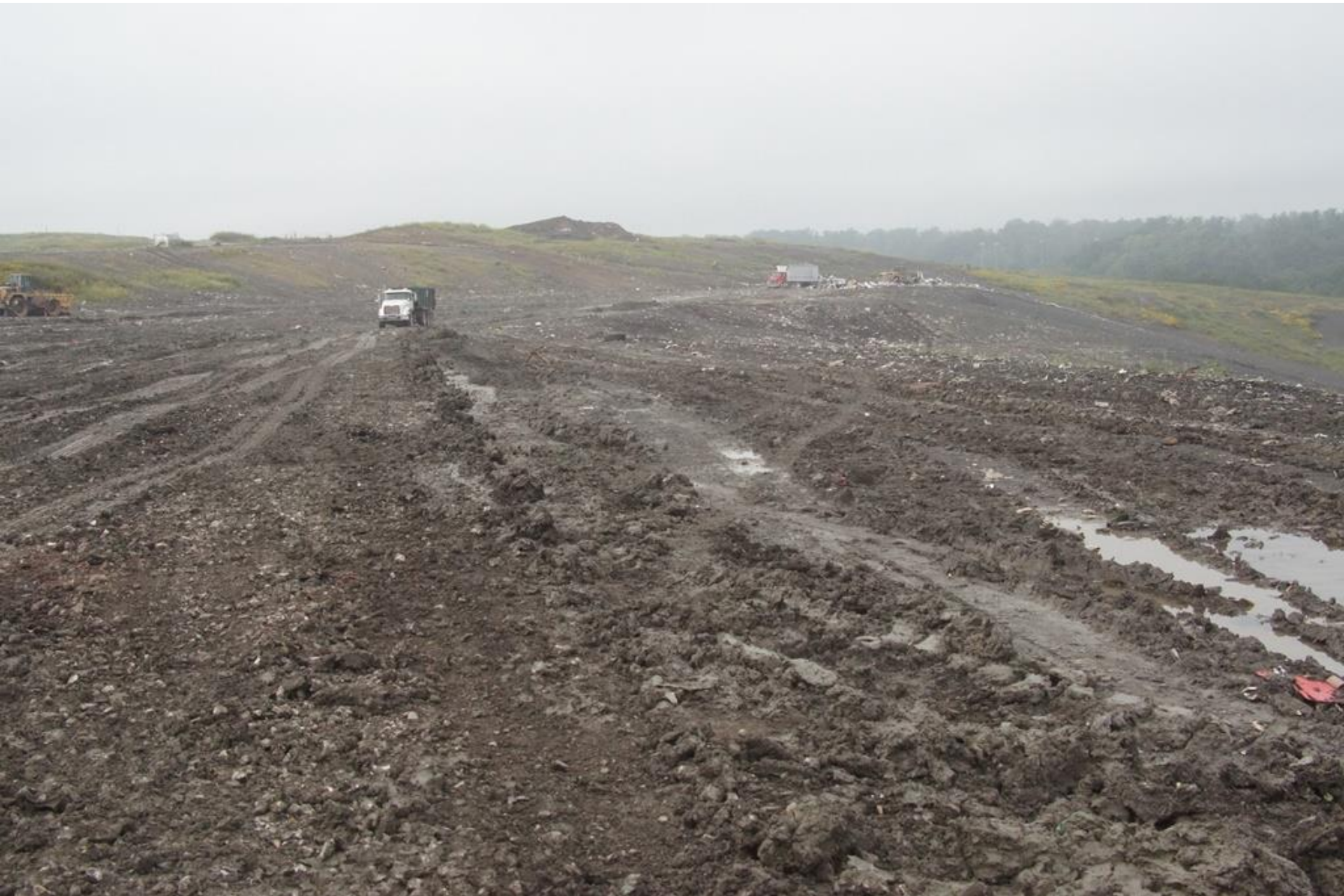
Advanced Disposal Blue Ridge Landfill AI 998 9/11/15 g. weems Muddy but trucks can still pass;
