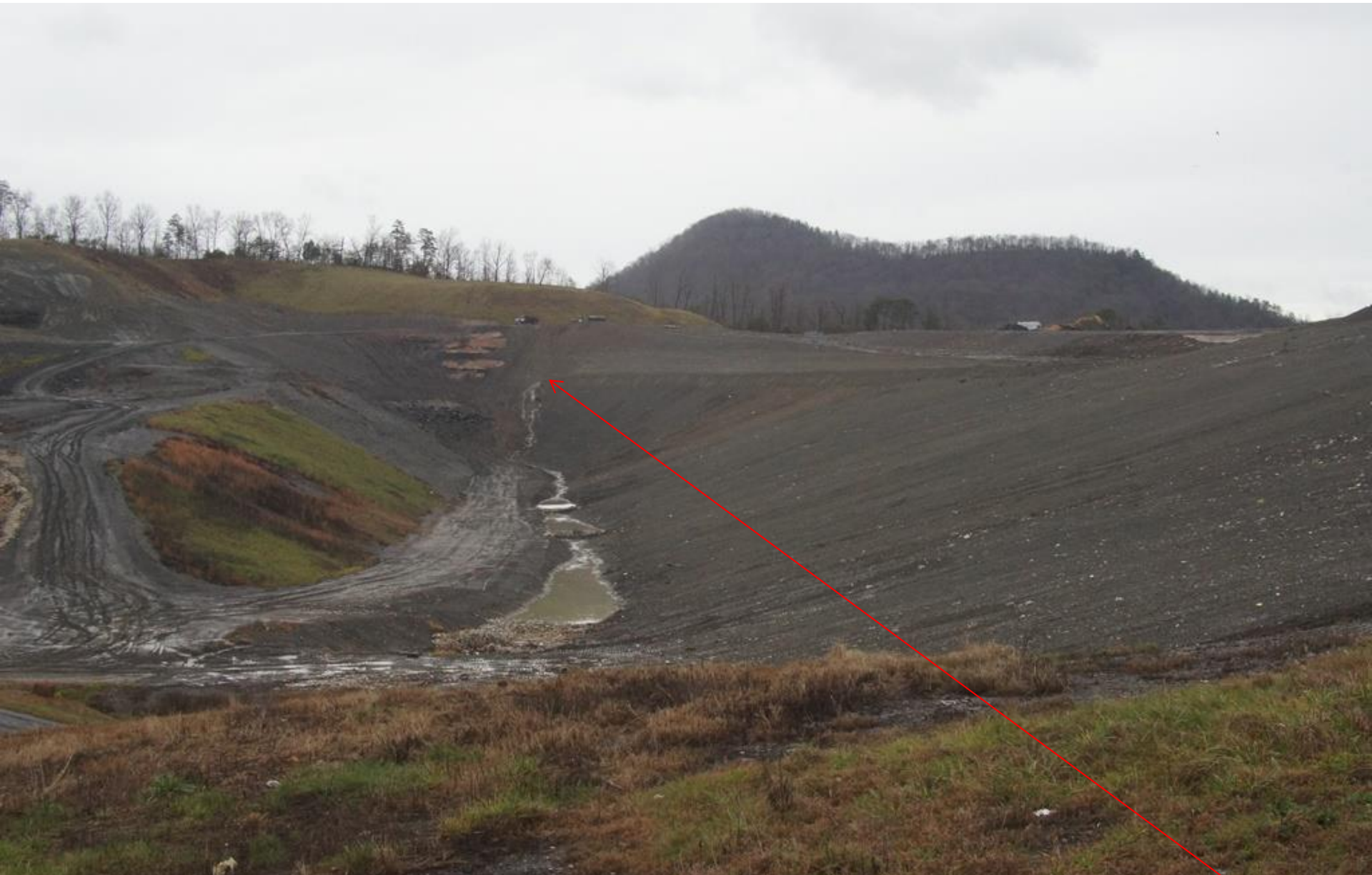
Advanced Disposal Blue Ridge Landfill AI 998 12/1/15 g. weems Rain is channeled to this point on the landfill to minimize the area being maintained.
