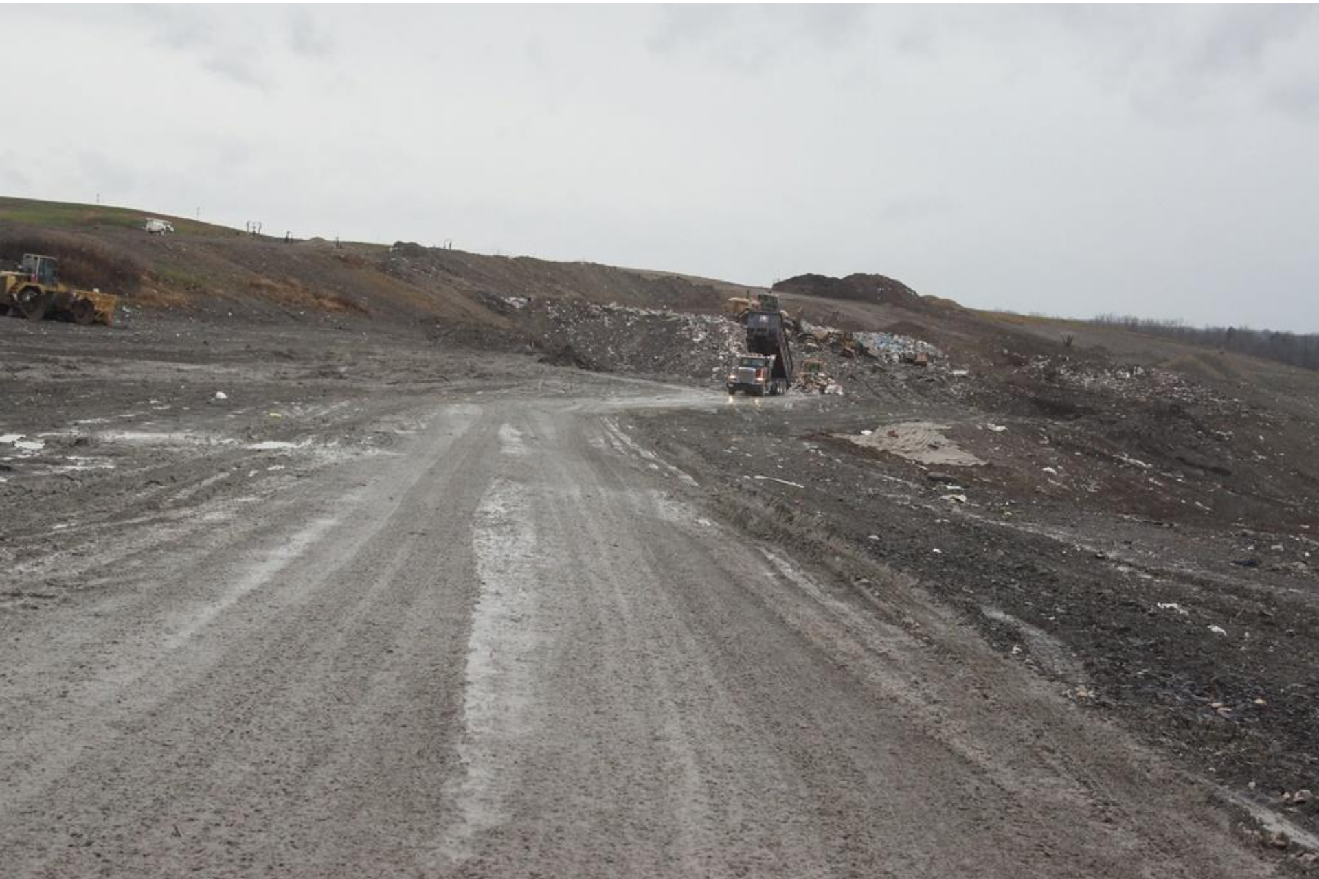
Advanced Disposal Blue Ridge Landfill AI 998 12/1/15 g. weems Working face.
